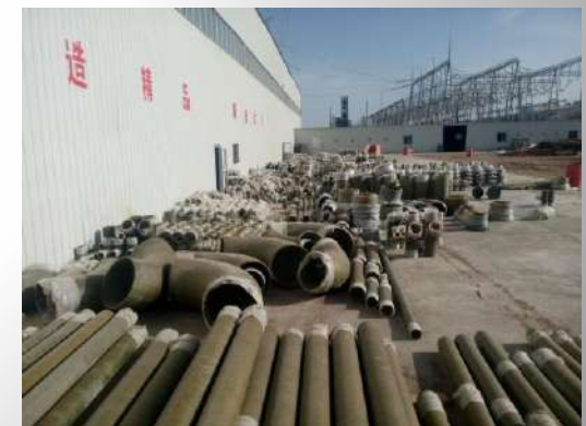
On site installation
